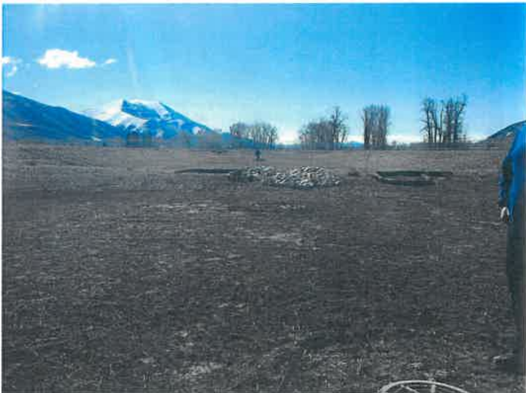
Drainage swale at S end of airport; 3 southern drywells appeared dry
