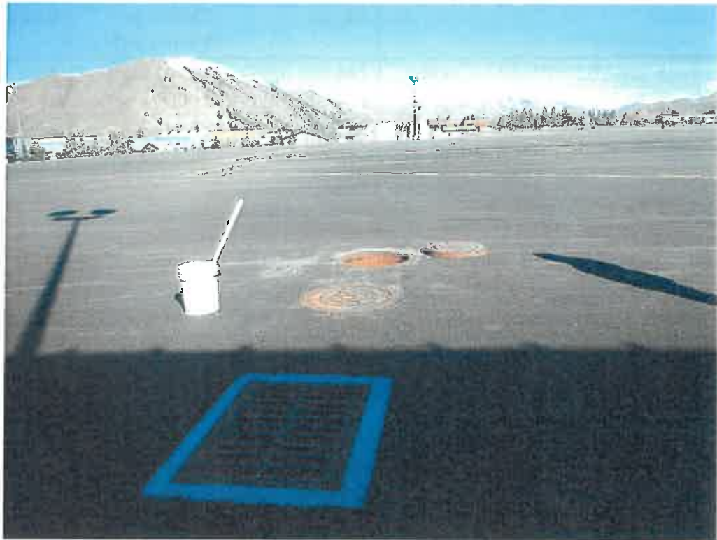
Manhole covers accessing drainage tank where de-icing fluid drainage flows
