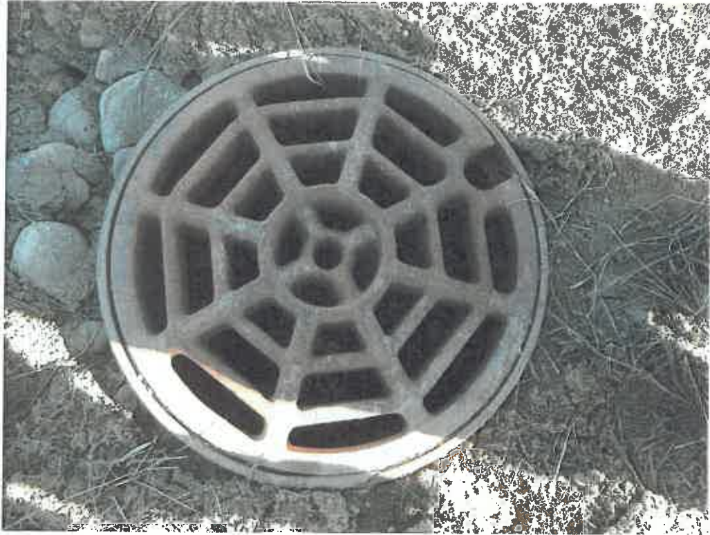
Northern most drywell in drainage swale; liquid is present
