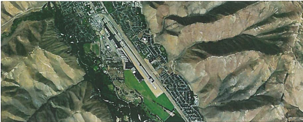
Figure 1. SUN Runway 13/31 and Immediately Surrounding Terrain
