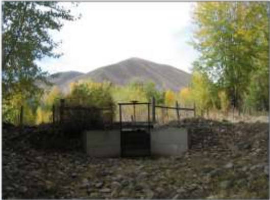
Photograph 2. POD for Rockwell-White Power Plant Canal, view northwest (Digital Image # 058)
