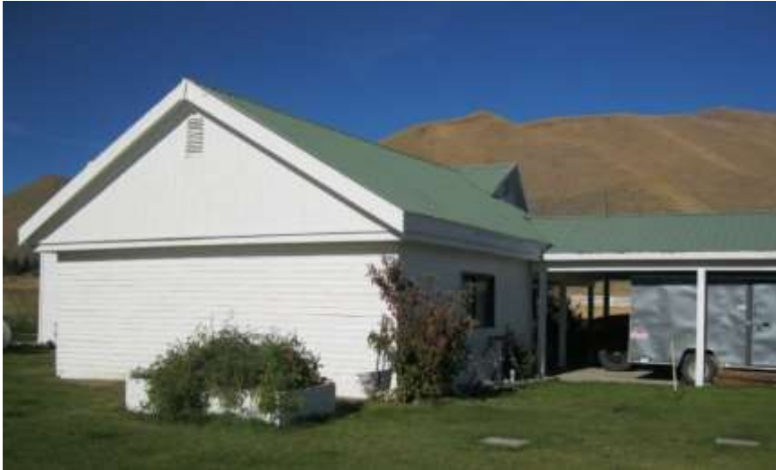
Photo 3. Detail of south and east elevation on the contributing farmhouse, view facing northeast.
