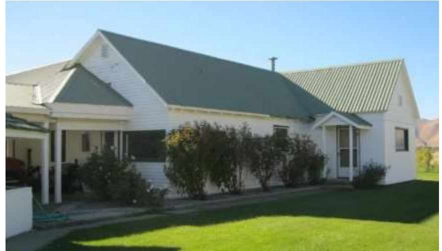
Photo 2. Detail of east elevation on the contributing farmhouse, view facing northwest.
