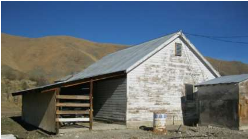
Photo 7. Contributing equipment shed, view facing northeast.
