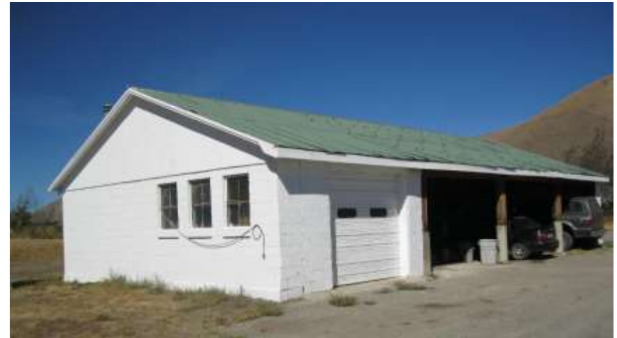
Photo 8. Contributing utility building and grain bin (roof visible in background), view facing northeast.
