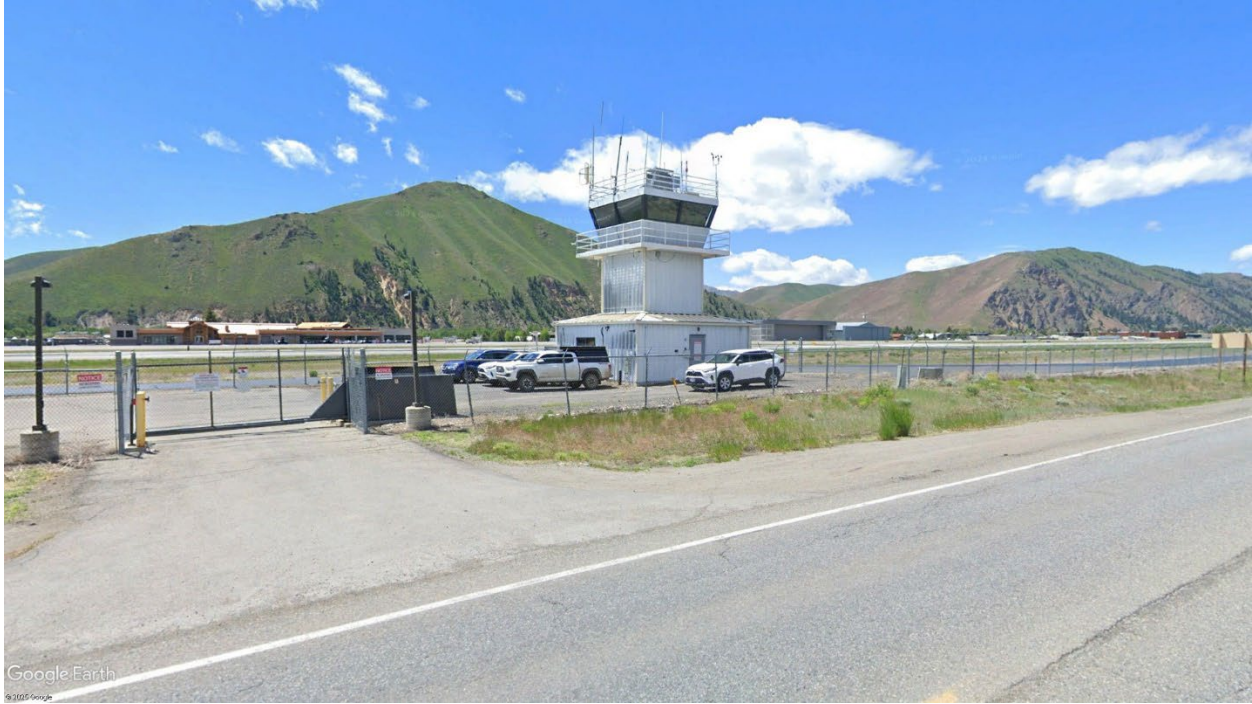
Figure 1-2 Photo of Existing ATCT at SUN
